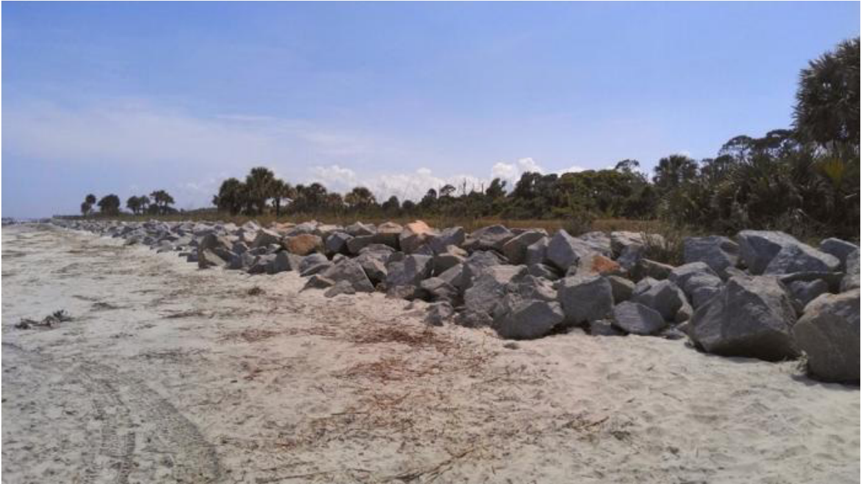
Rock Structures along the upper shoreline, designed to prevent land loss
